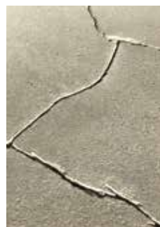
Initial State of Floor
