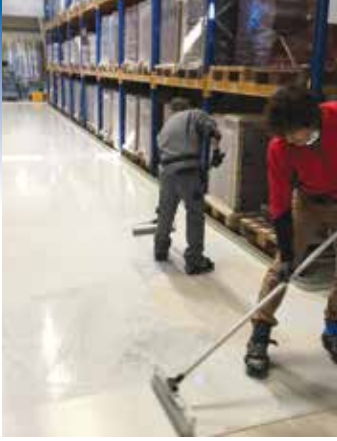
Applying the Top Coat
